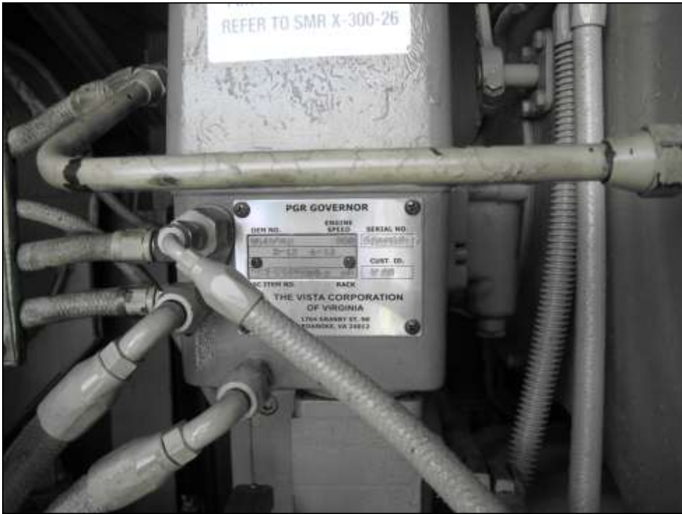
Mechanical engine governor ID.
