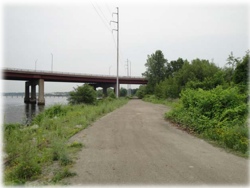
Pre-construction looking toward Dexter Rd, Henderson Bridge (New Red Bridge) and Seekonk River visible in the background
