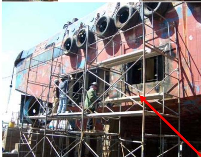
Modified keel cooler pocket
