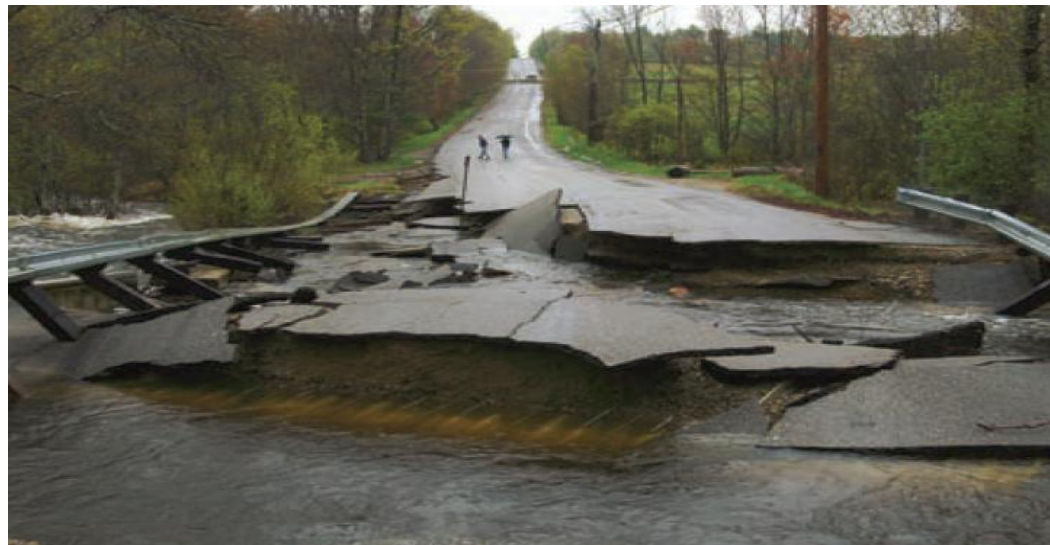
Culvert Failure
