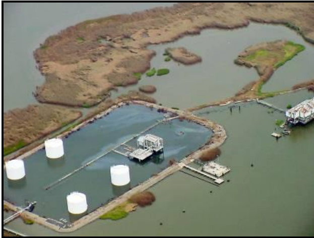
Inundation & corrosion of infrastructure
