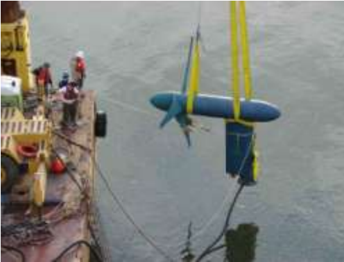
Verdant Power axial flow turbine
